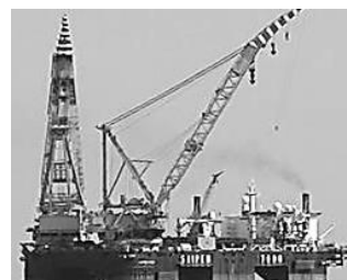
Drilling platform outside from Larnaca port
